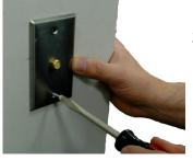
2. Mount the wall plate onto the wall in the area to be monitored.
